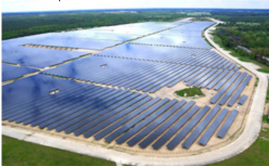
Alt Daber PV plant
